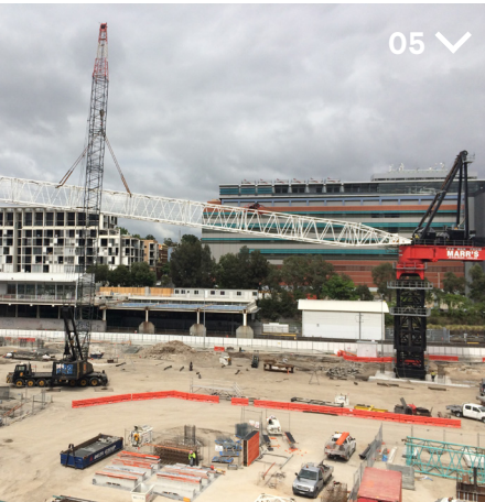
The boom being installed on the M2480D tower crane.
