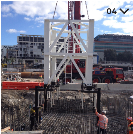
In June 2014, the first crane base was installed.
