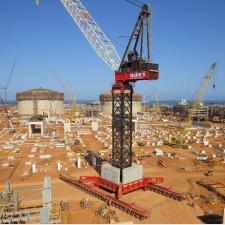
OCTOBER 2013 – NOVEMBER 2016 (Barrow Island): The SMPT trailer solution we used to load the M2480D onto Miss Hannah was employed at the LNG Plant to move tower cranes around the construction site within 1.5 hours instead of taking 2-3 weeks to dismantle and reassemble each time a crane was relocated.
