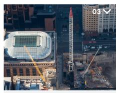
Excavating on a congested CBD site in the middle of a busy pedestrian thoroughfare and high traffic area presented a number of challenges for JHCPBG, including lifting 14 plunge columns that were 30-metres long and weighing 80 tonnes each as well as the associated 90-tonne drilling rigs, excavators and spoil removal.
