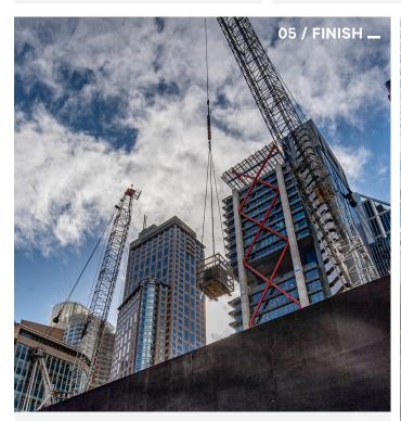
Use of the 150-tonne capacity M1280D allowed for the 80-tonne plunge columns to be prefabricated offsite and lowered into their final position – eliminating the need for complex technical welding of smaller sections on-site. This was a more efficient and safer solution which helped JHCPBG to deliver the Martin Place South site ahead of schedule.
