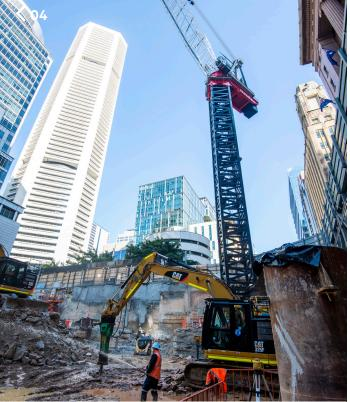
With a challenging schedule of works, JHCPBG partnered with Marr for a better solution to the original scheme proposed which relied on crawler cranes operating from a platform over the site and on the street, which would have required costly and risky road closure permits. Our solution was to eliminate the need for road occupancies by installing one of our M1280D heavy lift luffers to do all the lifting from a single point within the site.
