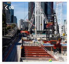
Flanked by Sydney Harbour, a rockface and another development to the south, the already congested site posed significant access and mobility issues for JHCPBG. The originally proposed craneage scheme was to use multiple mobile cranes and a 600-tonne capacity crawler, but was inefficient in such a congested space.
