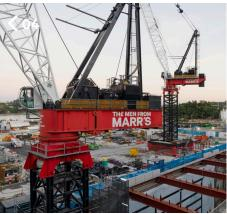
Marr's solution was to install one of our M2480D and M1280Ds sitting alongside the station boxes to provide lifting capacity across the project. Set on purpose-designed foundations in and outside of the station box, the cranes took up 90 per cent less room than the proposed traditional crawler crane and gantry set up.
