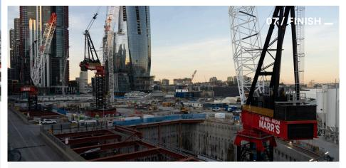
After the TBM was dismantled and transported offsite, the M2480D was reconfigured to continue general construction works on the project. Using Marr's higher capacity cranes gave JHCPBG the option to build with precast beams allowing for increased modularisation and fewer lifts. Marr's approach has also reduced congestion, improved site utilisation, and reduced complexity, risk and time on the project.
