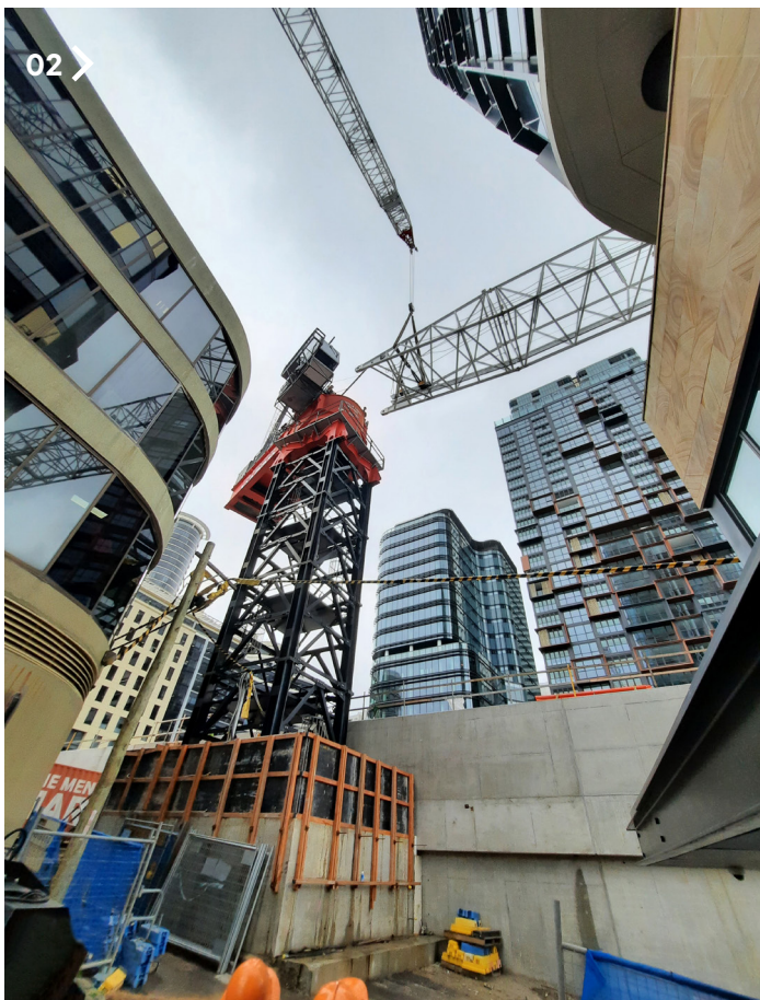
The area available to establish a crane capable of lifting precast elements weighing up to 150 tonnes across a 95m x 30m-wide rail cutting was just 7m wide. By installing one of our M2480Ds on a bespoke compact piled foundation with a 64-metre boom, Marr's solution provided our client, Arecon, with the unique combination of the M2480D's heavy lifting capacity and small footprint (equivalent to two passenger cars parked side-by-side).
