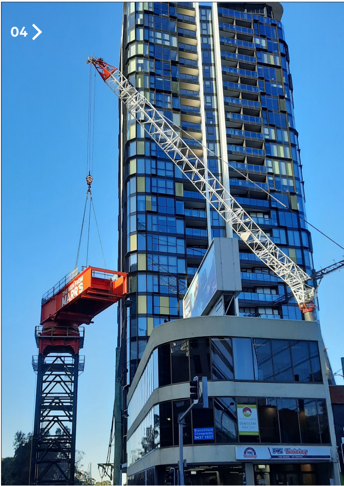
The limited space and tight access also proved a challenge for Marr's construction team and rigging crew during the installation and removal of the M2480D using our Grove GMK6400 mobile crane.
