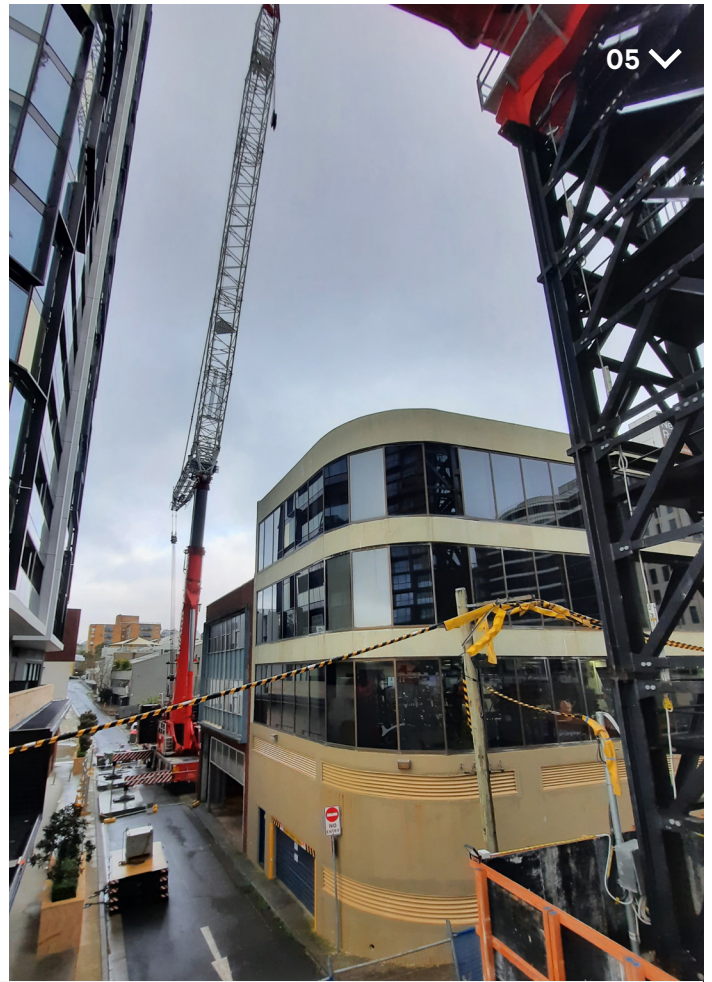
The limited space and tight access also proved a challenge for Marr's construction team and rigging crew during the installation and removal of the M2480D using our Grove GMK6400 mobile crane.
