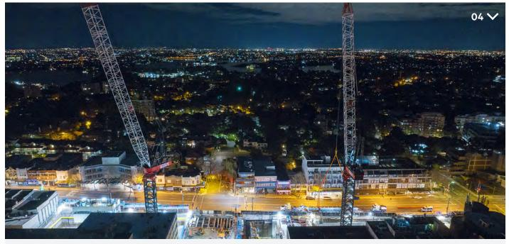
Marr's solution – using two M2480Ds installed within the station box — provided the heavy lifting capacity required within the small space available within the construction site.
