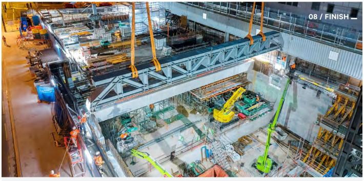
With a lifting capacity of up to 330 tonnes, the M2480Ds allowed large, heavy components such as steel truss beams to be fabricated off site and installed in single lifts, eliminating the need for temporary works.
