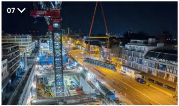
Installing heavy lift luffing cranes within the station box also addressed the logistical challenges that came with the lack of space available for the delivery of materials to site and the handling of large precast and steel elements weighing up to 120 tonnes.
